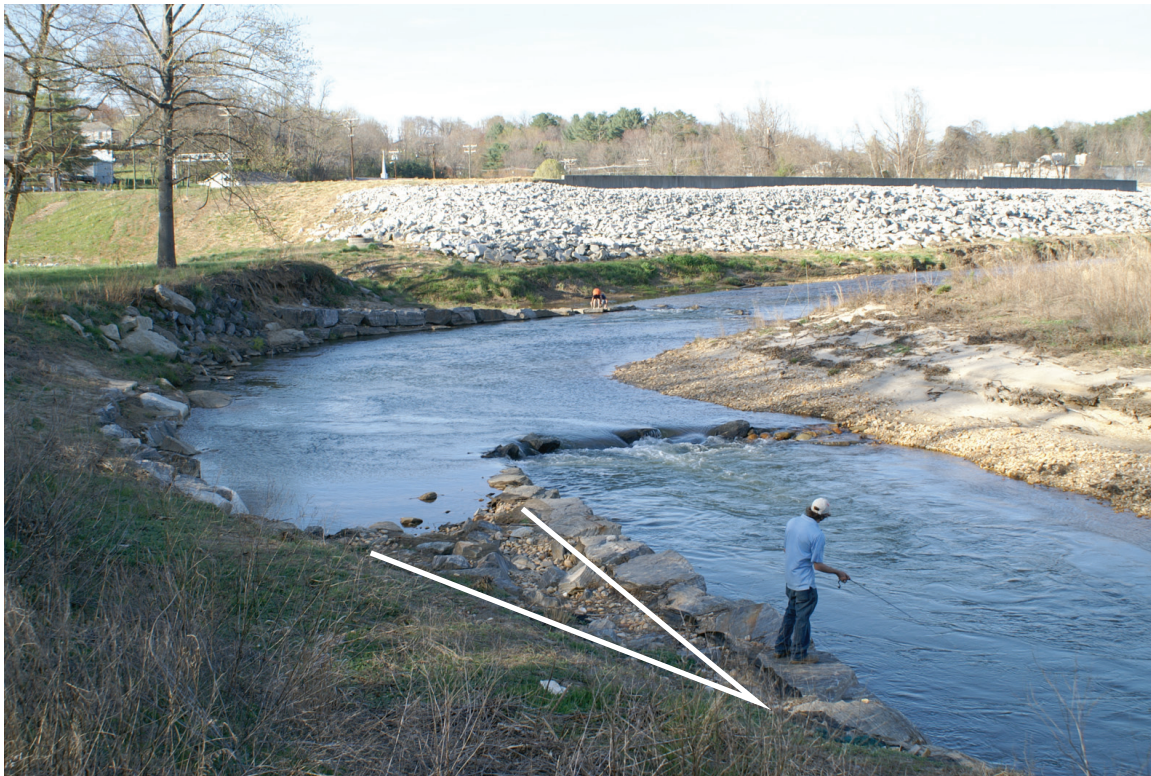
FIGURE 11: J-HOOK VANE AT BASE FLOW. The triangle is formed from the vane arm where the fisherman is standing and the streambank. The structure is placed downstream of where the velocity vector intercepts the bank.
