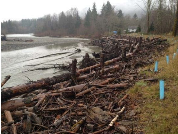
Figure 36: Complex timber revetment (photo credit: Tim Abbe, USBR and ERDC 2016).
