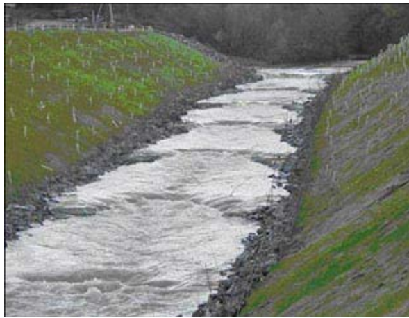
Figure 40: Pool and weir fishway.
