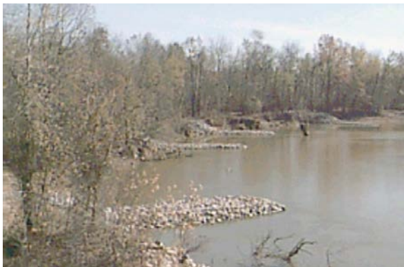
Figure 49: Bendway weir (Lagasse et al. 2009).
