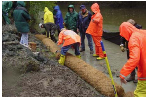
Figure 51: Installation of coir fascines (NRCS 2007, TS14I).
