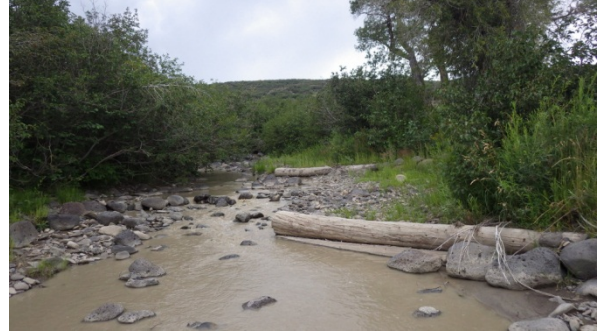
Figure 47: Log vanes at low flow providing bank stabilization and channel narrowing 2 years after construction (Milk Creek, Colorado).
