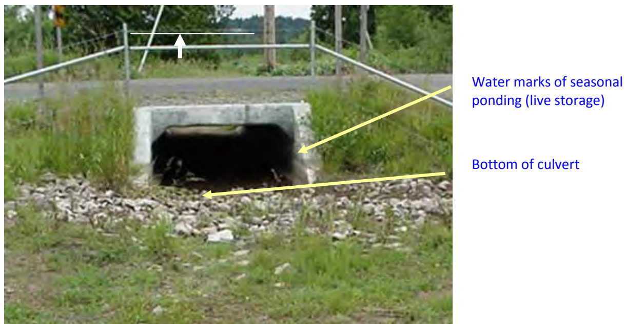
Figure24: A box culvert that is the outlet of a depressional wetland. The live-storage is measured as the distance between the bottom of the culvert and the water marks on the side. The distance here is approximately 15 inches.
