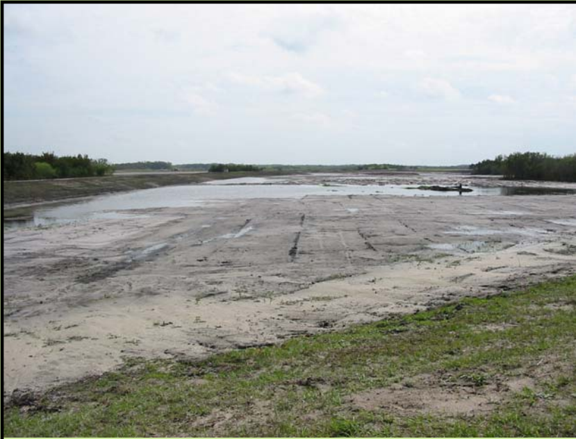
Recently constructed wetland, showing NO topographic relief (MTB).
