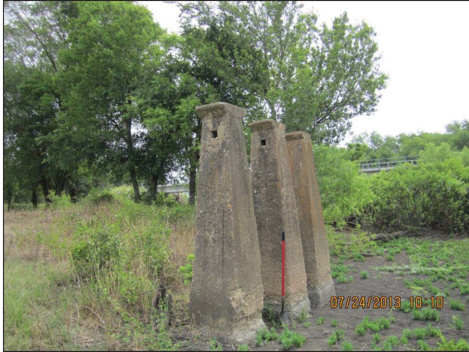
Figure 13. View of the railroad piers looking downstream with the Chambers Creek scar to the right. Note the 4-inch-square holes in the upper part of the two closer piers.
