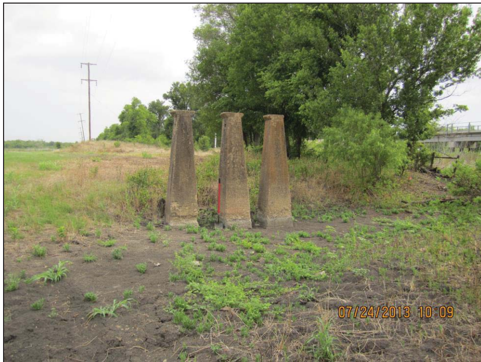
Figure 12. Concrete piers that supported the Texas Electric Railroad crossing of Chambers Creek and was built before the creek was channelized. An earthen berm is north of the piers and the power pole is set into the top of the berm. View is to the north.
