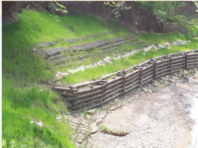
Live Cribwall – Pottawatomie Co. KS
