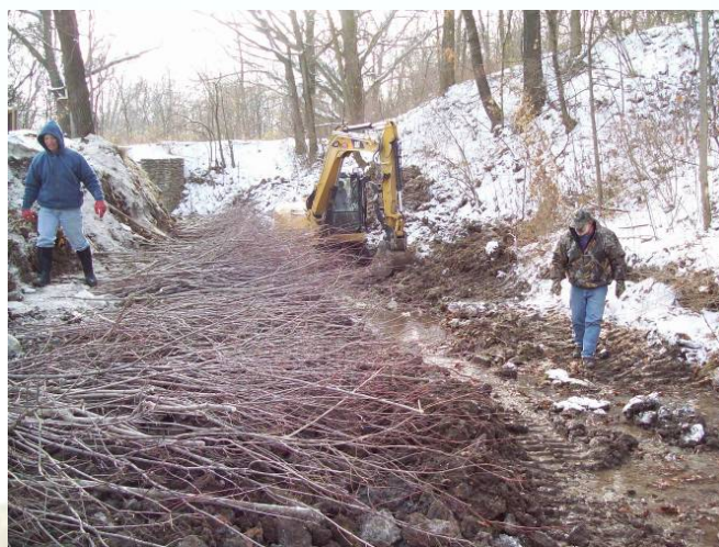
Phil Balch -Vegetated Geo-grid Installation– Wyandotte Co. KS
