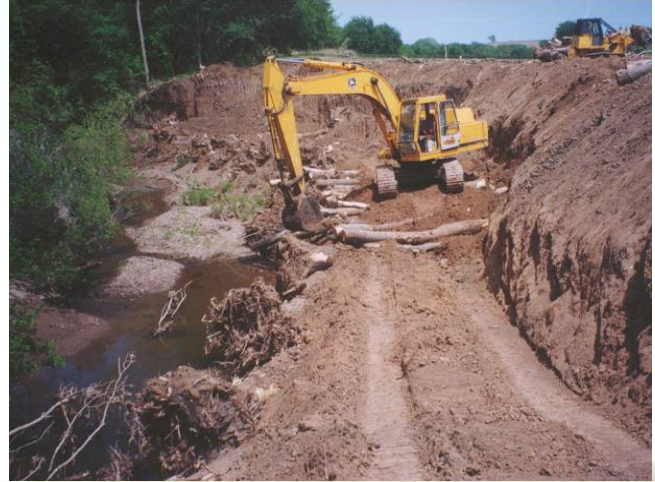
LWD – Root wad Stabilization – Sharps Creek – KS
