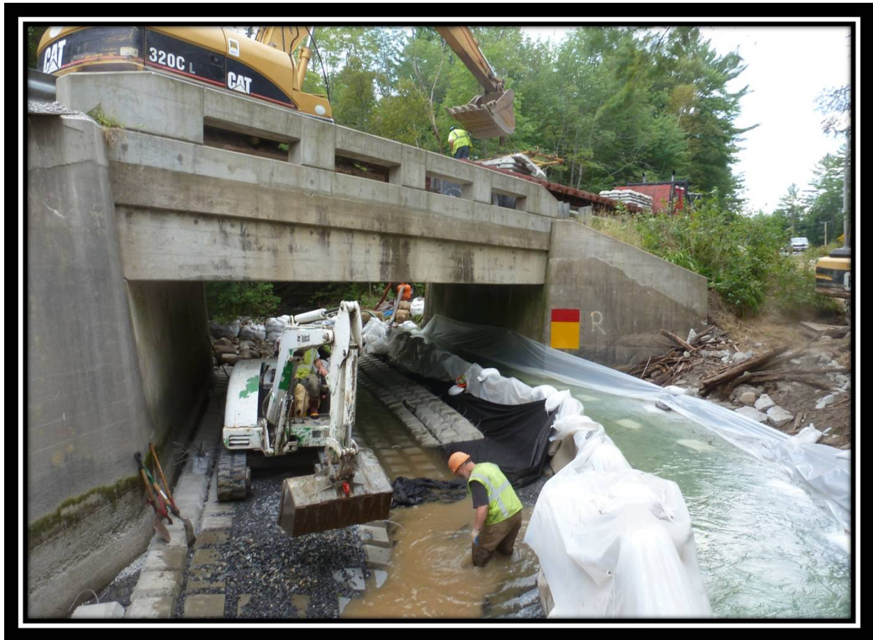
Figure 3-30. Concrete cable mat installation. A migratory pathway will be maintained throughout the construction process in situations where stream width will allow.
