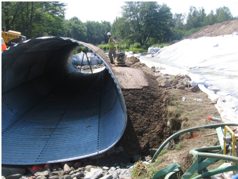
Figure 3-19. Bedding a corrugated metal culvert.
