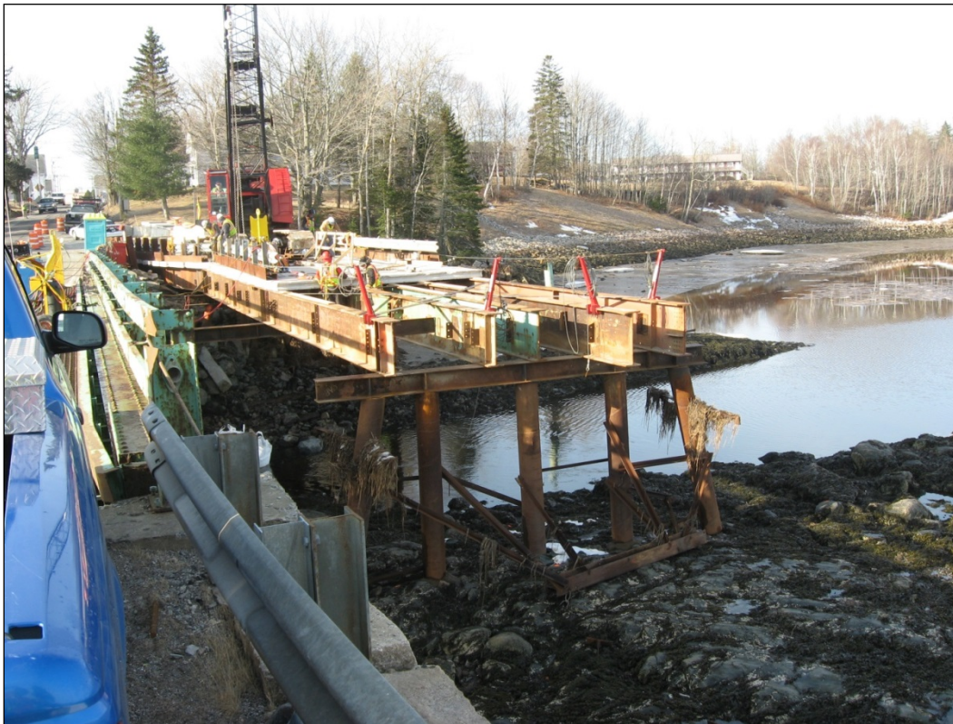
Figure 3-35. Typical trestle/temporary bridge construction.
