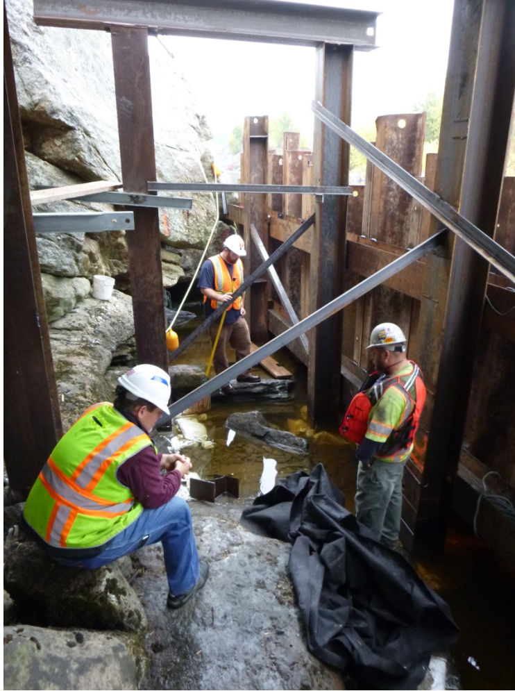
Figure 3-22. Example of the inside of a sheet pile cofferdam used for abutment construction on a bridge replacement project.
