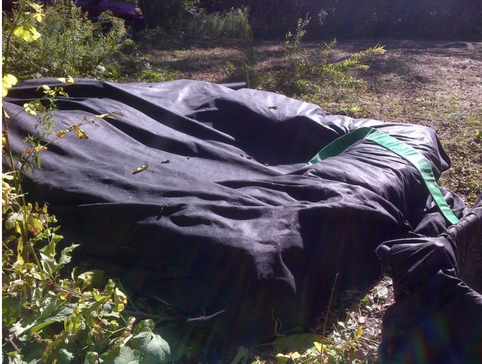
Figure 3-14. Hay bales and geotextile fabric used as part of a dirty water treatment system.
