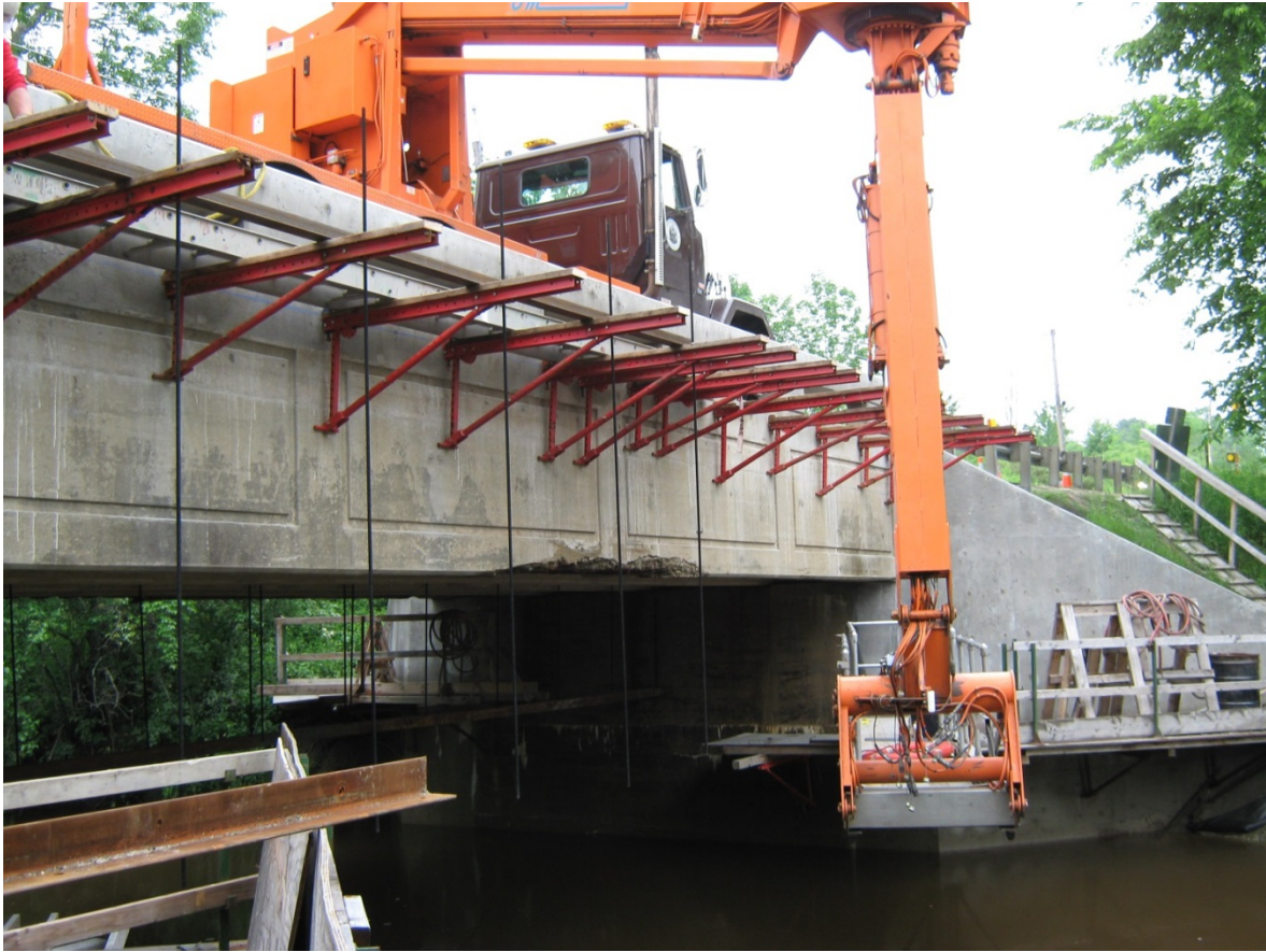
Figure 3-34. Concrete repairs on beams will be completed from staging. In this photo, the staging is attached to the wing wall.
