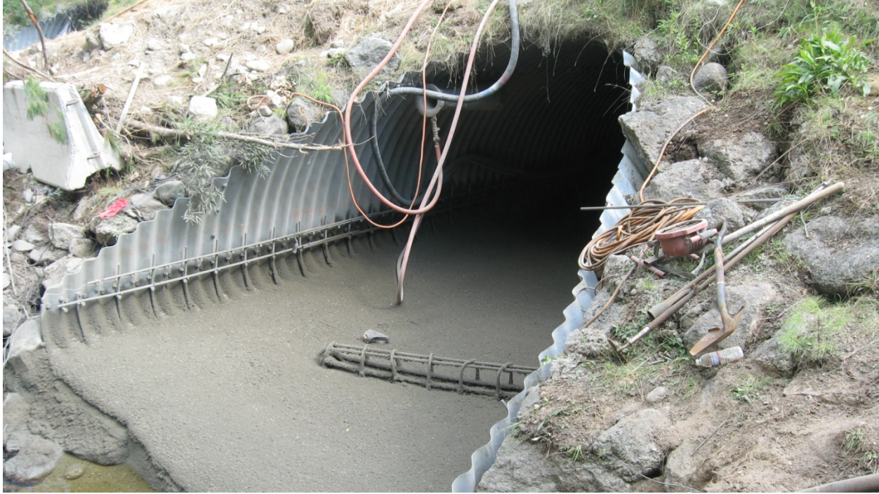
Figure 3-37. Concrete freshly placed during an invert lining. Note the rebar cage for fish weir support.
