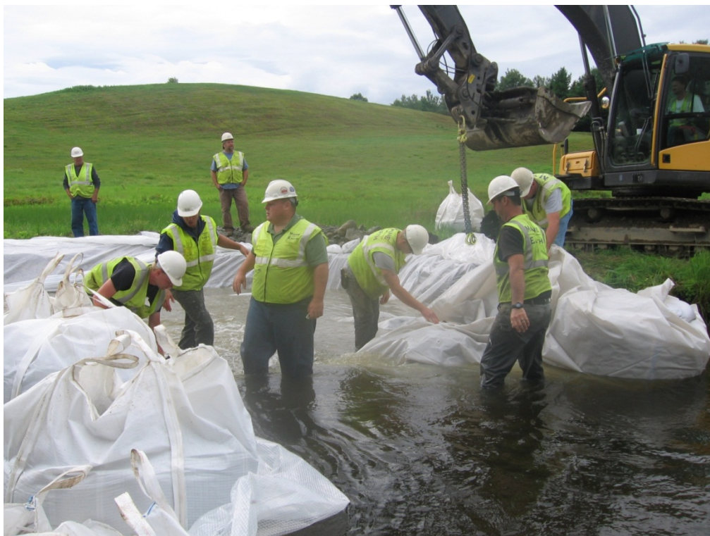
Figure 3-3. Placement of plastic sheeting under sandbag cofferdam.
