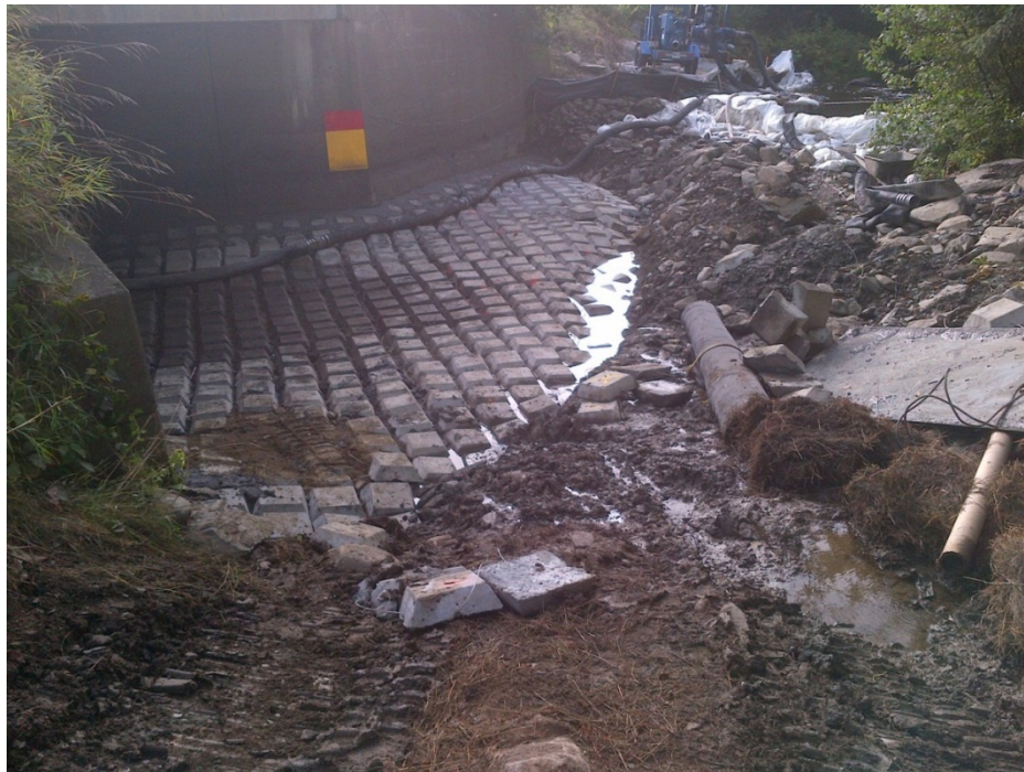
Figure 3-31. Concrete cable mats “toed in” on the upstream edge of a bridge.
