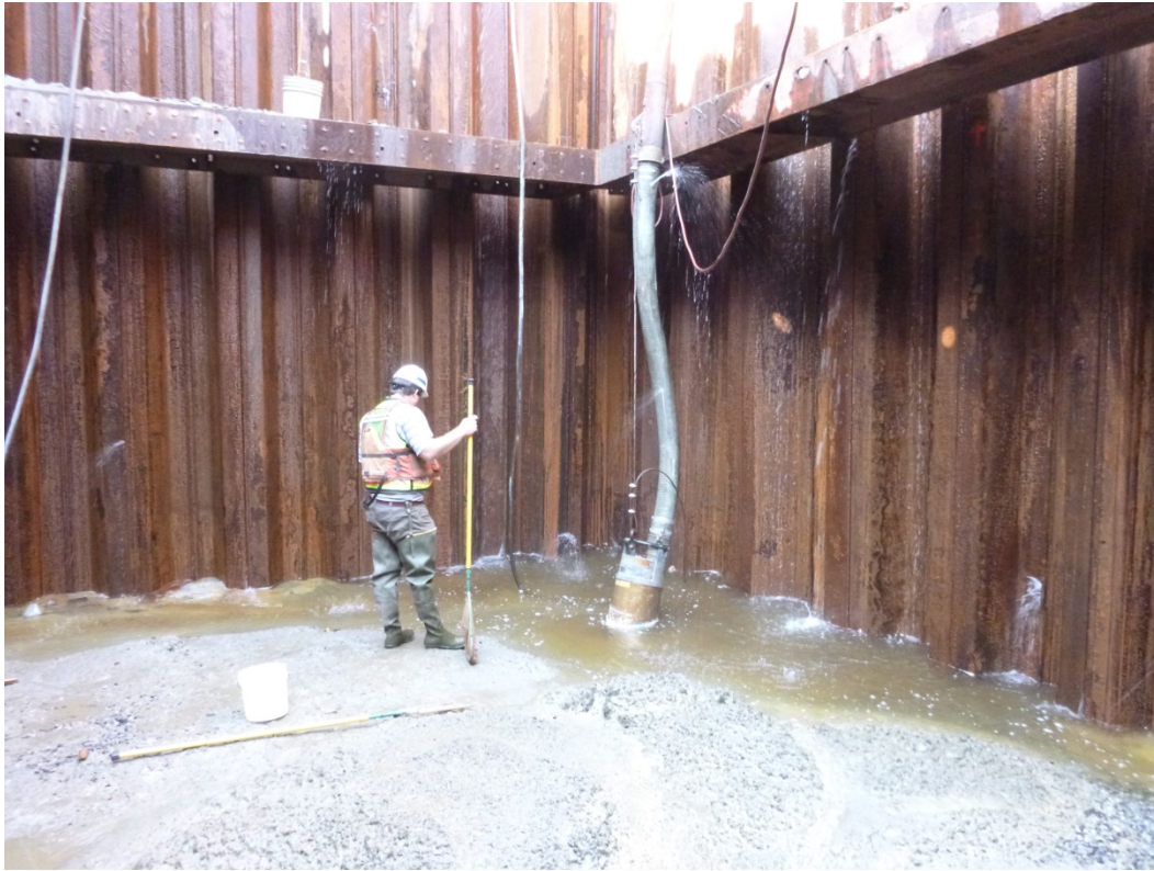
Figure 3-24. After excavating the substrate, concrete is poured across the entire bottom inside of the sheet pile cofferdam to create a “dry” work area for constructing the pier. A maintenance pump is still necessary for maintaining the “dry” conditions.
