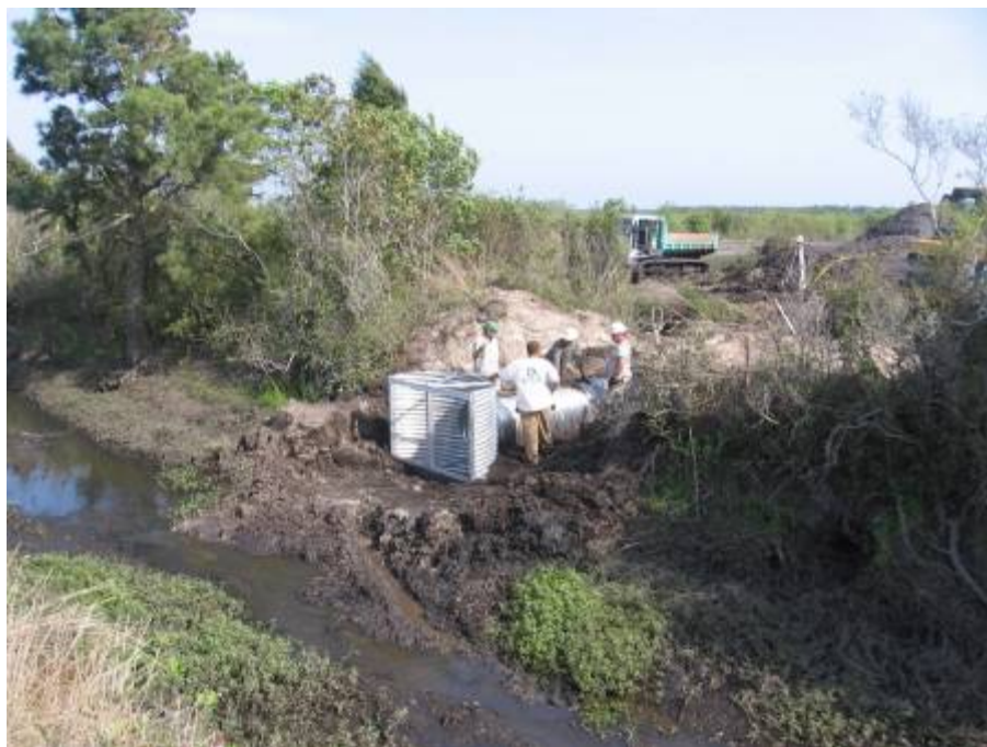
Figure 26. Installation of the water control structure that feeds the freshwater portion of the restoration (Summer 2007)
