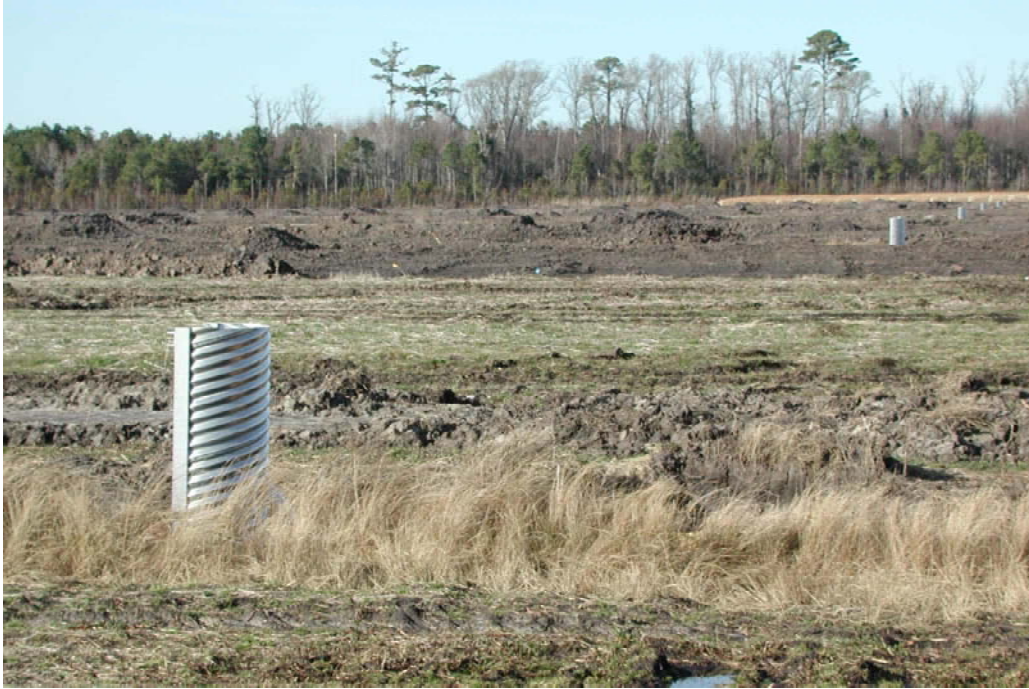
Figure 5. Water control structures (flashboard risers) shortly after installation (Winter 2003)
