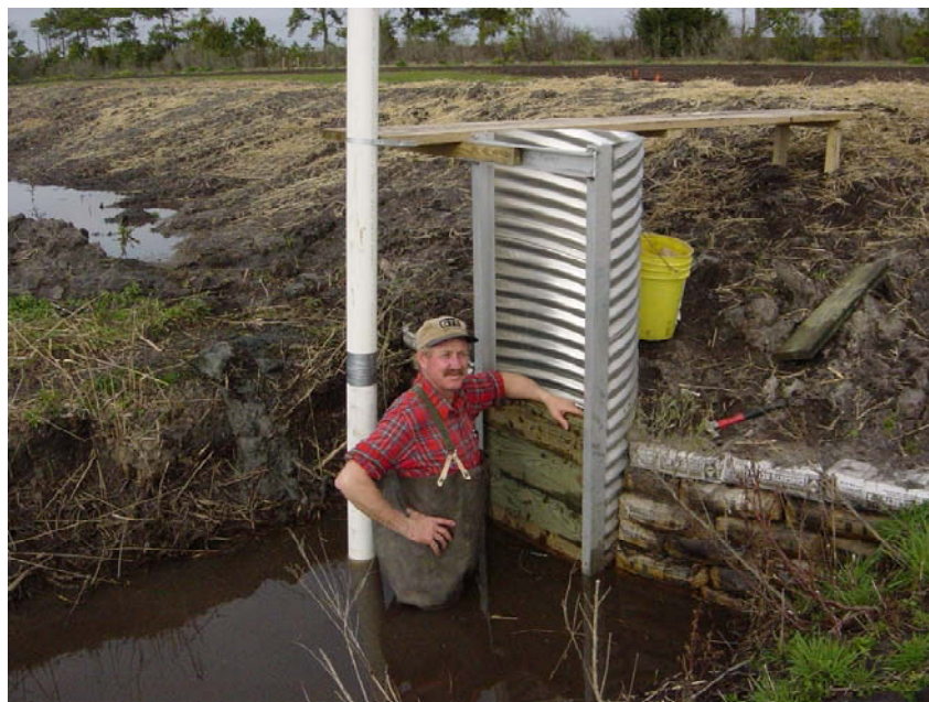
Figure 6. Dr. Robert Evans installing flashboards that controlled outflow from the restored wetlands (Spring 2003)
