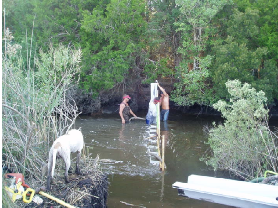
Figure 27. Installation of the low rock weir that diverted drainage water into the tidal marsh portion of the restoration (Fall 2007). Sheet piles were jetted into the canal and reinforced by marl. This design allowed for fish passage during incoming tides and during outflow events.
