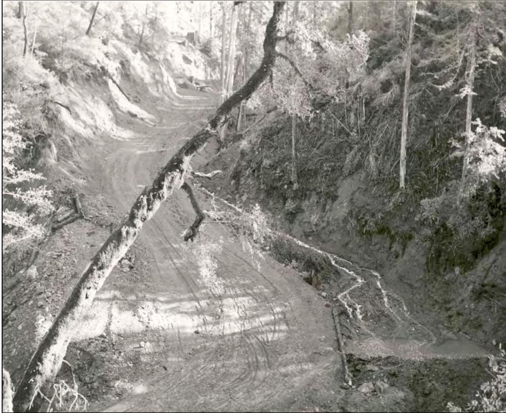
**Figure 1.** *This 1955 photo of Signal Creek tributary where heavy equipment operation has obliterated the riparian zone and stream channel and where a legacy of high erosion risk is in evidence (CDFG, 1955).*
