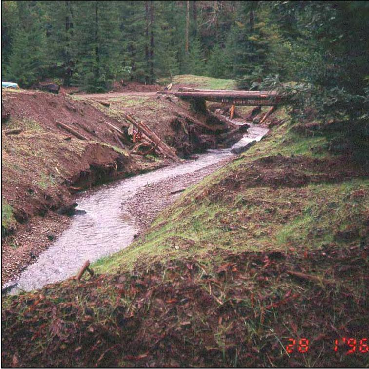
**Figure 2.** *“This photo shows a flatcar bridge spanning the channel of Olsen Gulch in the middle of a stream channel restoration project. The stream here was formerly disrupted by fill from a landing likely placed shortly after World War II. Jack Monschke directed excavation of 50,000 cubic yards of material and re-contoured the stream channel under contract to Coastal Forest Lands, Inc.” (KRIS Garcia, 2003.)*
