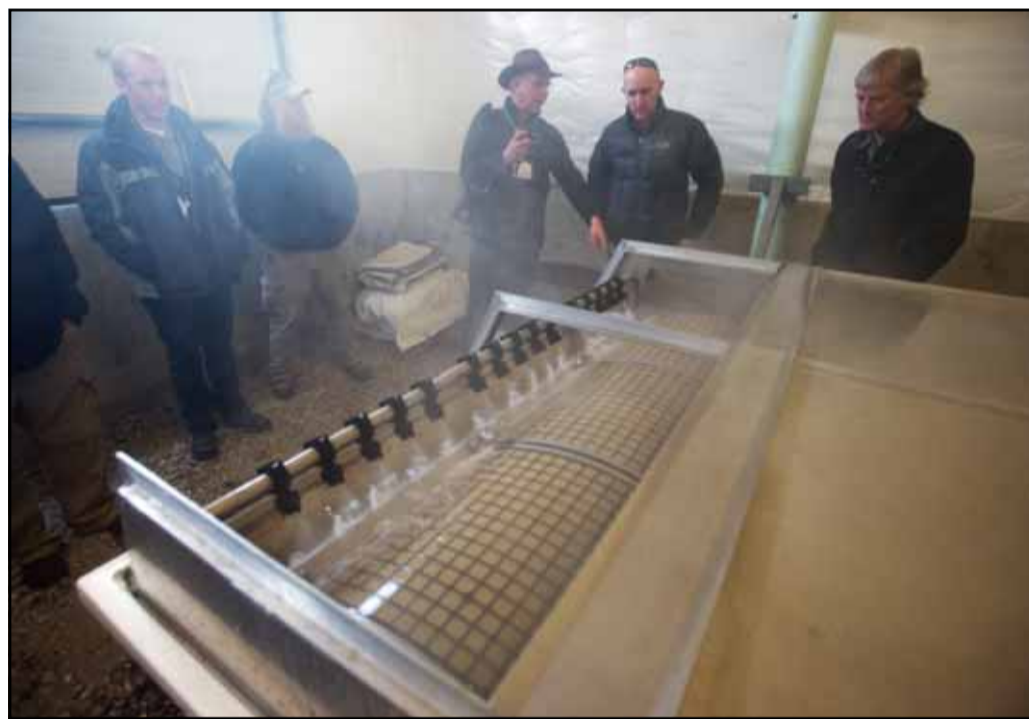
Water spray clouds the air as people on the tour watch how water sprays onto a drum filter, cleaning it.
