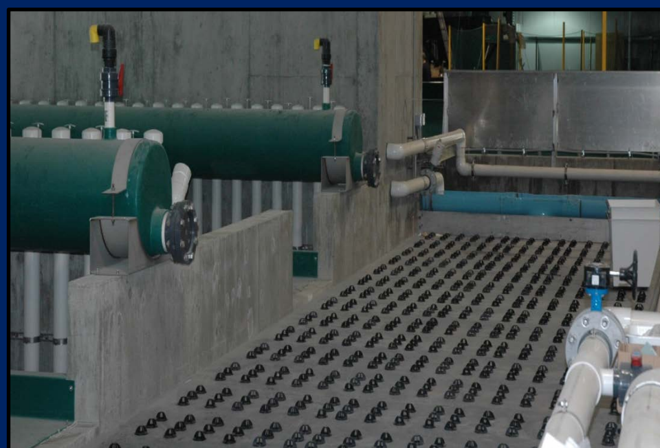
November 29th, 2012 Quarantine unit biofilter. Carbon dioxide strippers to the left.
