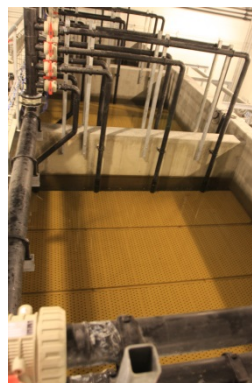
Biological filter – fixed bed filter – cleaning of filter Transformation of ammonia ( \text{NH}_4^+ ) to nitrite ( \text{NO}_2^- ) and nitrate ( \text{NO}_3^- ) (end product!!) Removal of organic material to carbon dioxide ( \text{CO}_2 ) and water
