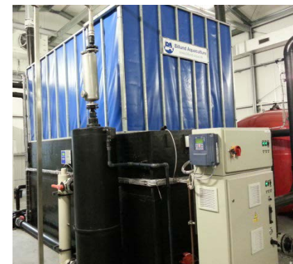
Removal of brownish colour by use of ozone
