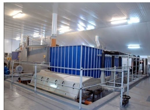
Trickling filter / Vacuum Degassing Removal of Carbon dioxide ( \text{CO}_2 ) and Nitrogen gas ( \text{N}_2 ) Aerating of water to approx. 100 % oxygen ( \text{O}_2 )
