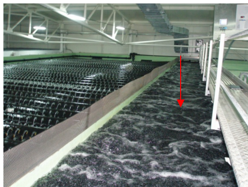
Biological filter – moving bed filter – no cleaning Transformation of ammonia ( \text{NH}_4^+ ) to nitrite ( \text{NO}_2^- ) and nitrate ( \text{NO}_3^- ) Removal of organic material to carbon dioxide ( \text{CO}_2 ) and water
