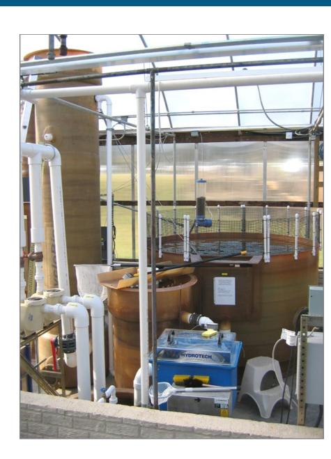
Ozone was added at the low head oxygenator (LHO) and monitored via Hach SC100 units with differential ORP sensors
