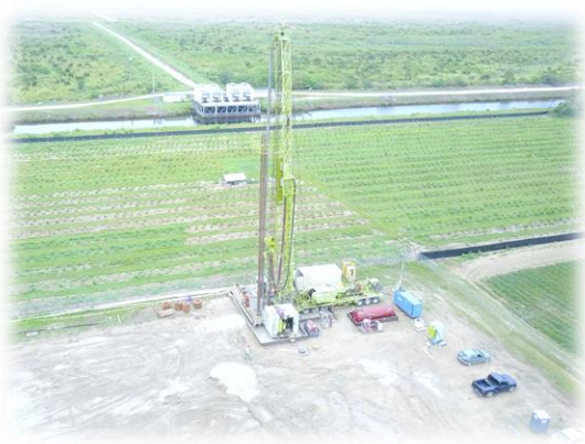
Mid-Floridan saltwater aquifer well drilling completed in September, 2017
