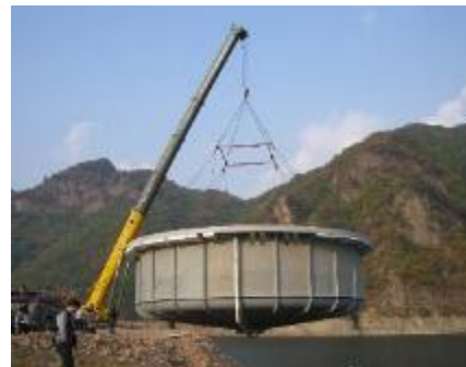
Tank installation
