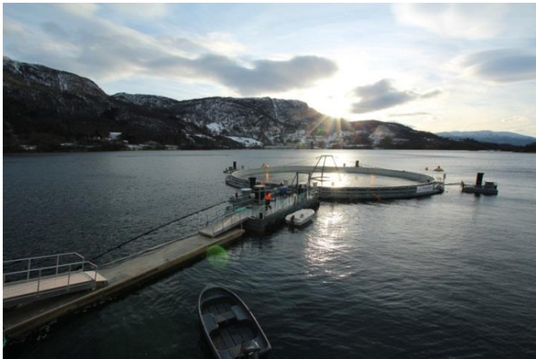
Floating semi-closed tank at Marine Harvest Norway site “Molnes”
