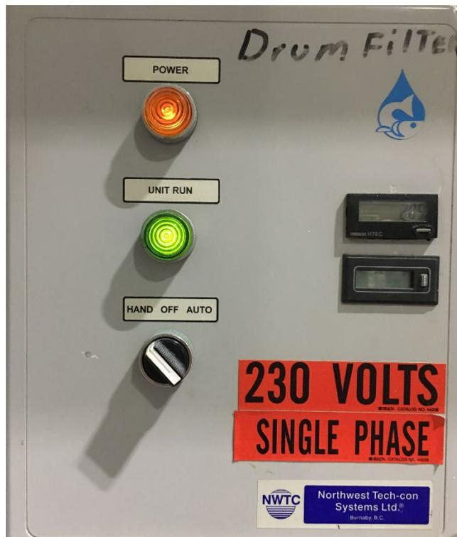
Figure 5. Drum filter control box. There is one HAND, OFF, and AUTO selector switch settings that controls both drum rotation and backwash spray.
