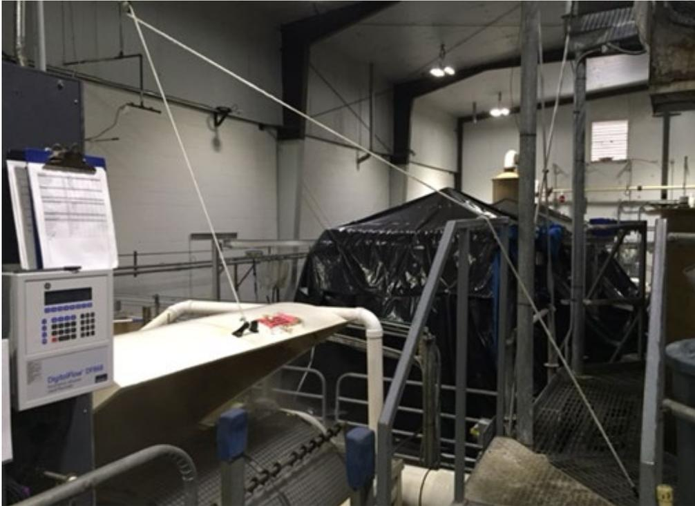
Figure 4. Properly opened and secured drum filter cover
